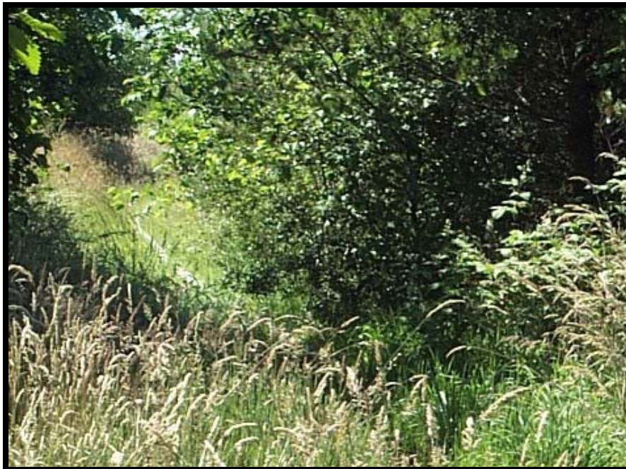
Operable Unit 1, Area 6. View of Area 6 groundwater extraction, treatment, and recharge system (grassed swale recharge area). Note the white perforated poly-vinyl chloride (PVC) discharge line.
