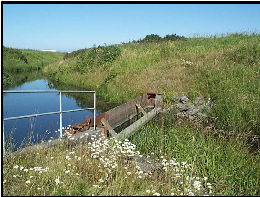
Operable Unit 3, Area 16. View of a portion of Area 16 that shows a “runway ditch,” the concrete baffle, and typical vegetation.
