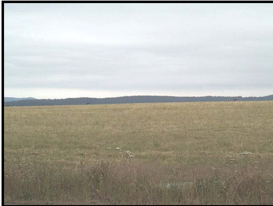
Operable Unit 1, Area 6. View of Area 6 landfill. Area 6 landfill is covered with a minimum functional geosynthetic cap with a vegetative cover. Note passive landfill gas vents in background.
