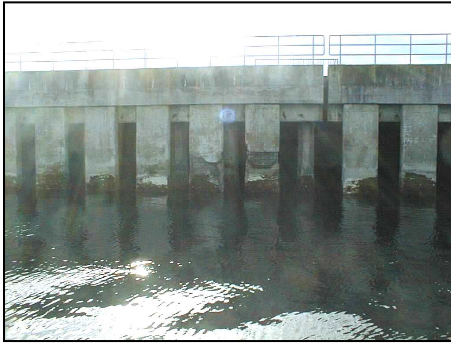
Figure 2-24. Pier B Wave Attenuation Baffles (Source: NAVFAC)
