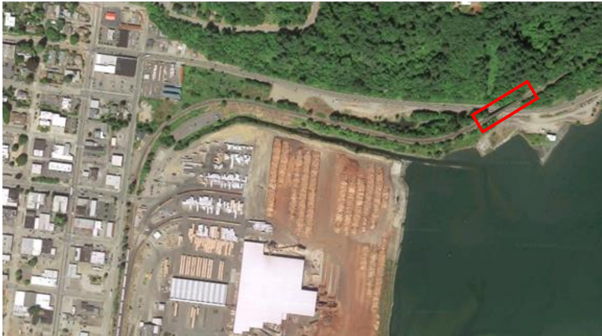
Shelton State Route 3 Bridge
