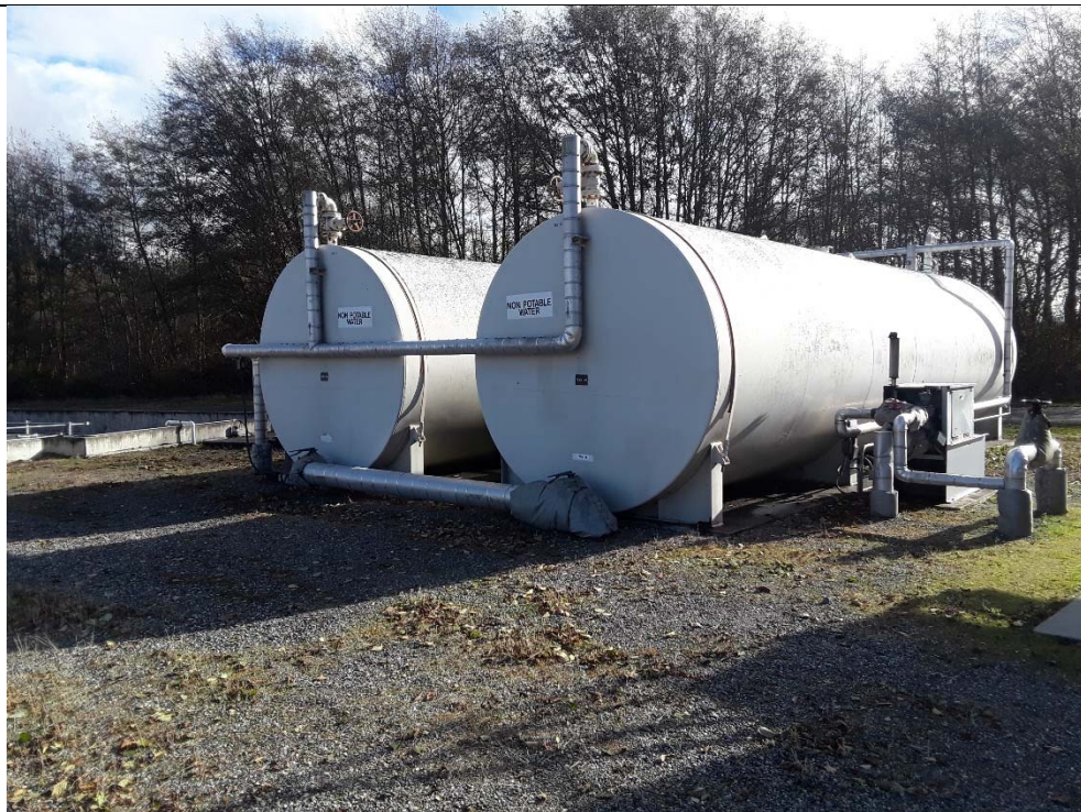
-Water storage tanks (all water used onsite is stored and recycled) (facing southeast)
