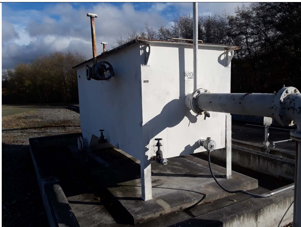
-Aboveground oil/water separator (facing southeast)
