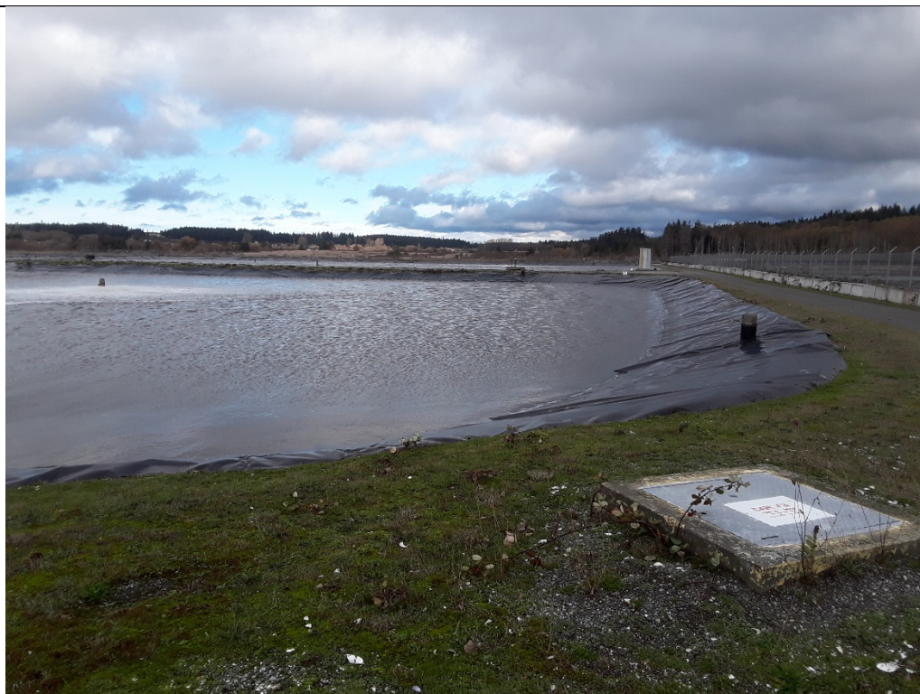
-Lined sewage lagoons (From southeast corner facing North).
