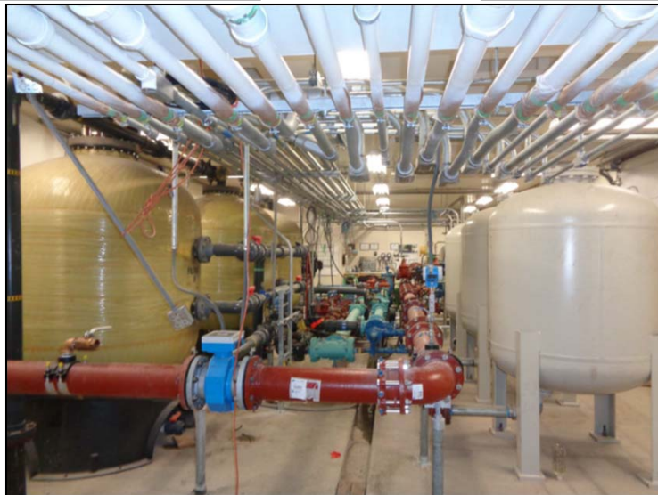
Inside existing WTP with new pipe, electrical conduit, and hydropneumatic tanks (photo to left)
