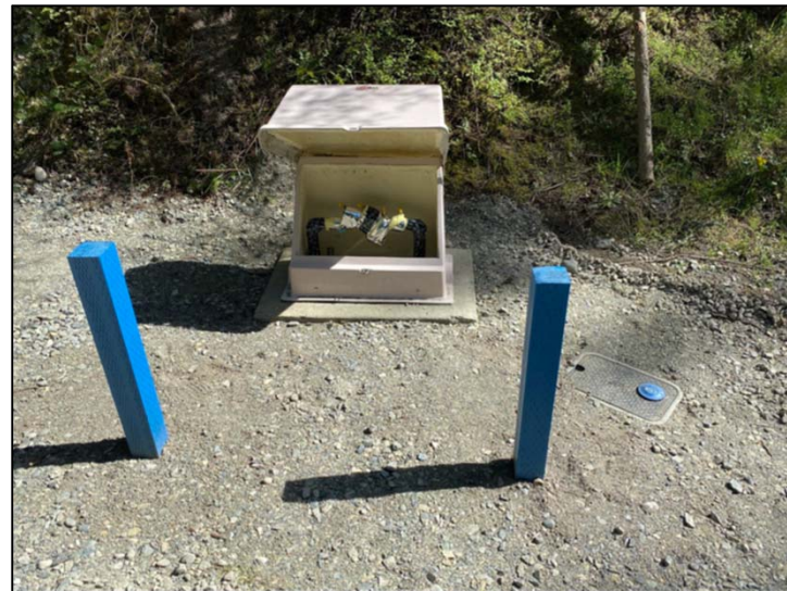
Backflow preventer and water meter at service line connection (photo to left)
