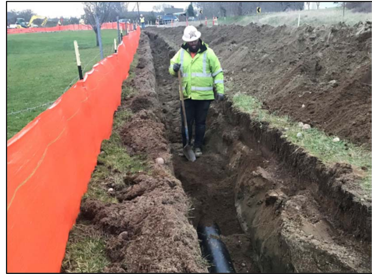
Placing new water main on State Route 20 (photo above)
