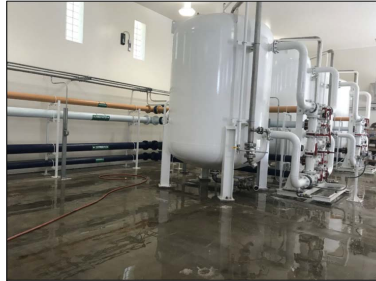
Inside new WTP with new granulated activated carbon vessels and pipe (photo above)
