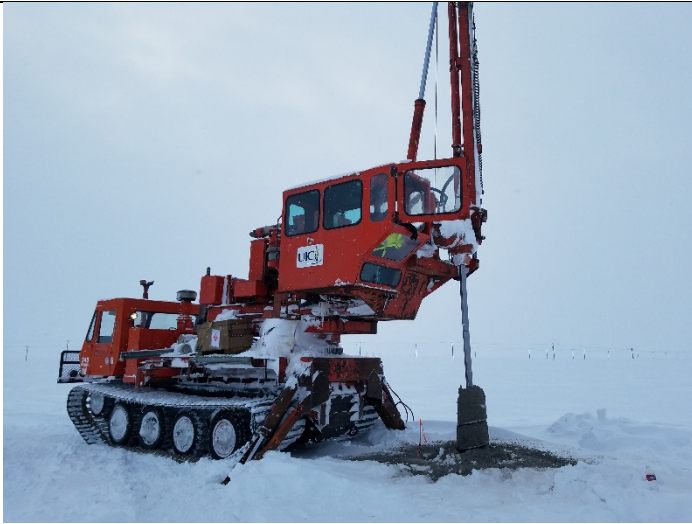
Drill rig pulling up soil core at Location 5 (Looking West) 13 March 2018
