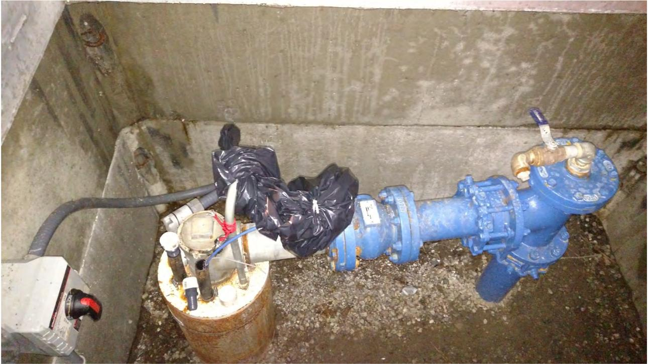
Transducer installed at Keystone Hill well—12/21/2017
