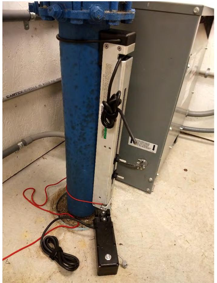
Ultrasonic flow meter installed on vertical pipe segment at Keystone Hill well pumphouse—12/21/2017
