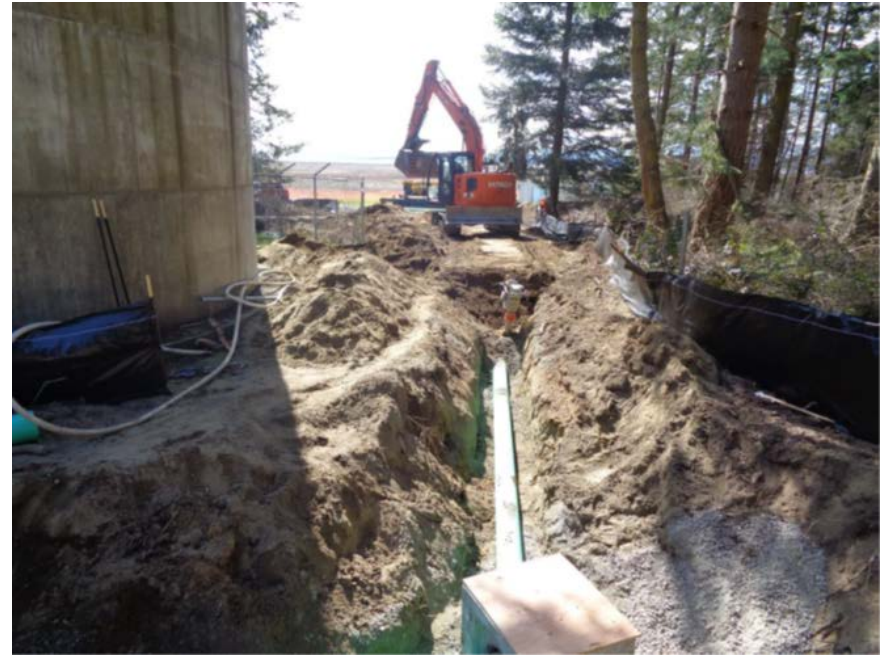
New storm drain lines (view south)
