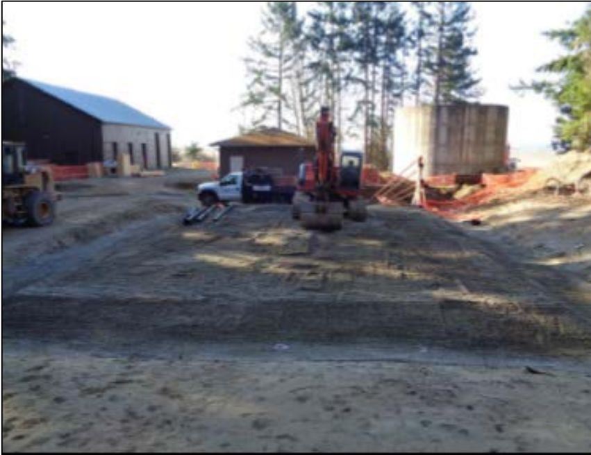
Subgrade preparation (view south)
