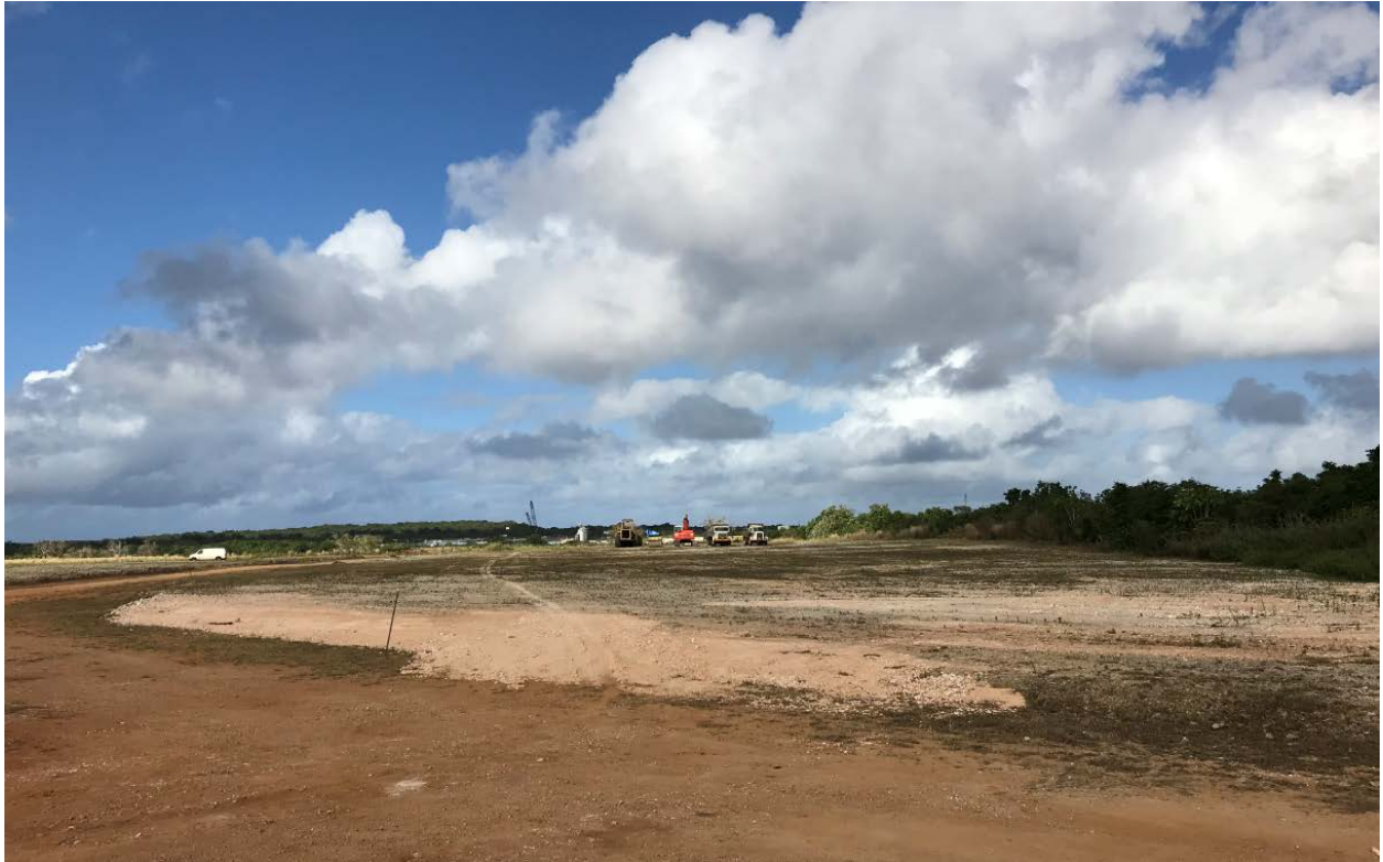
Figure 2. Recent clearing and grading at the proposed laydown area.
