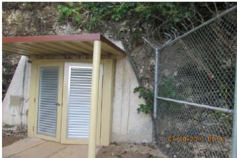
Rehabilitated Entrance to Tunnel
