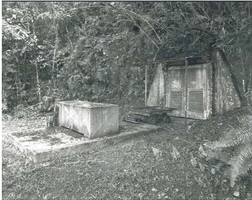
Entrance to Tunnel
