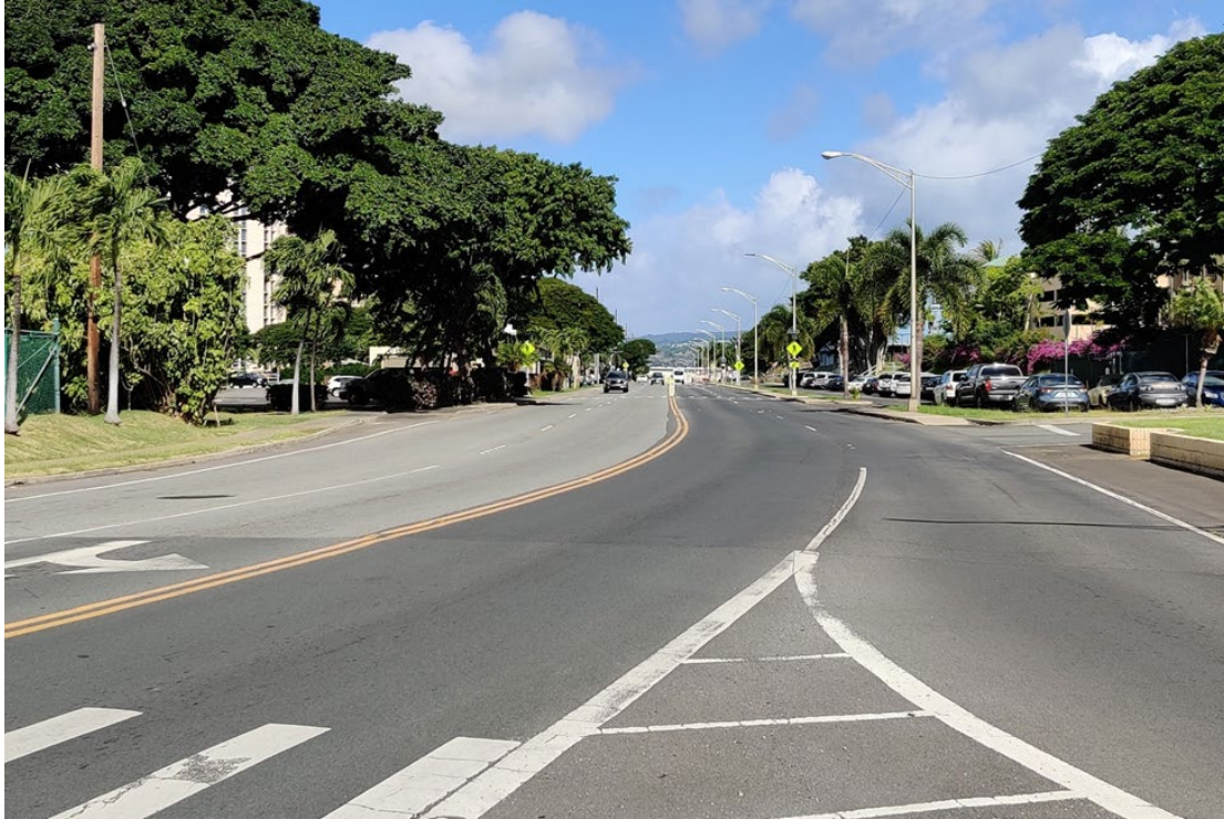
Photo 3.7-1. RRFBs along North Road.
