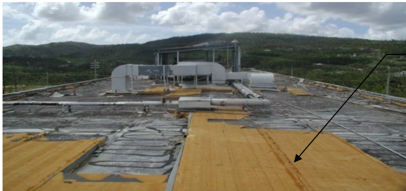
Figure 17: Typhoon Damaged Roof Insulation
