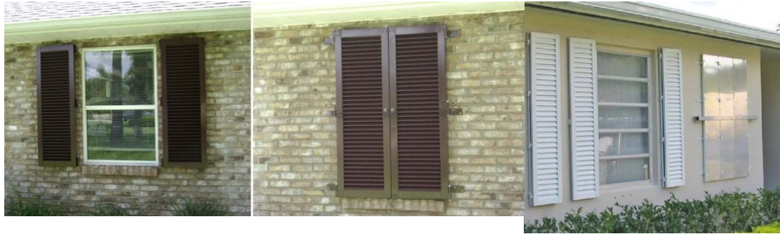
Figure 7: Typhoon Shutter Side Hinged
