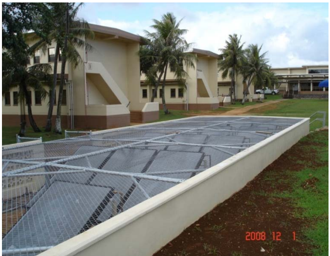
Figure 19: Solar Panel Enclosure
