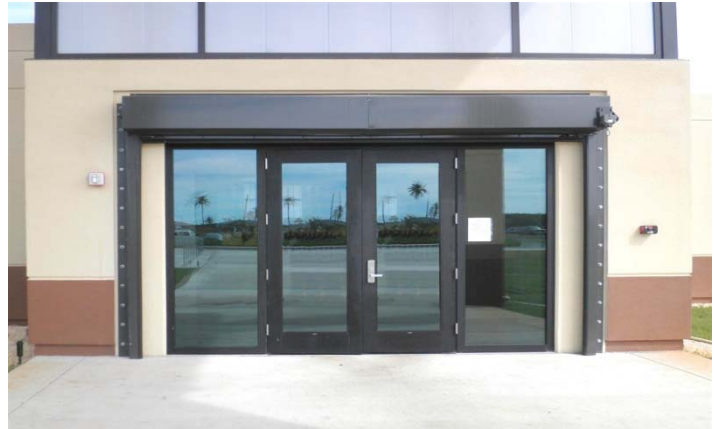
Figure 13: Typhoon Shutter Add-on Example
