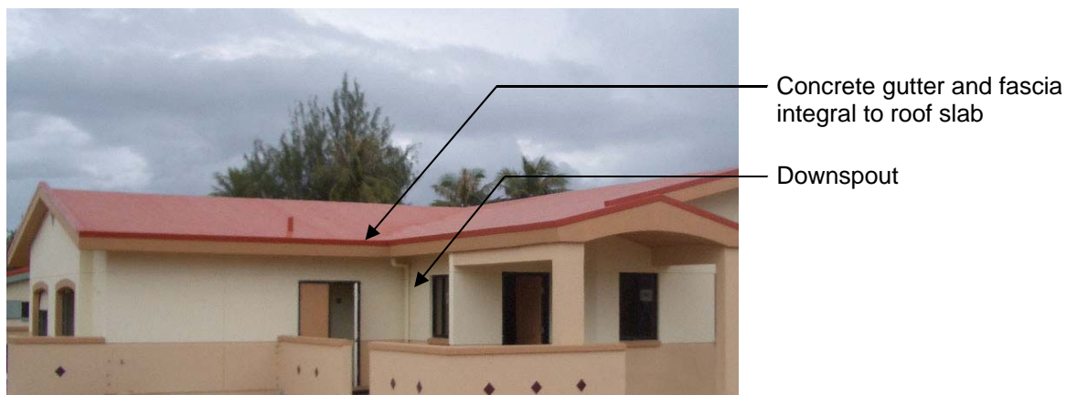
Figure 18: Integral Concrete Gutter and Fascia
