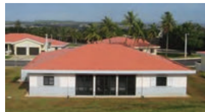
Fluid applied roof coating on hip roof; see Building Color chapter for acceptable roof colors
