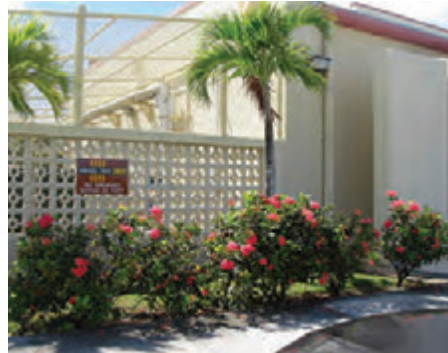
Layered planting softens the equipment enclosure
