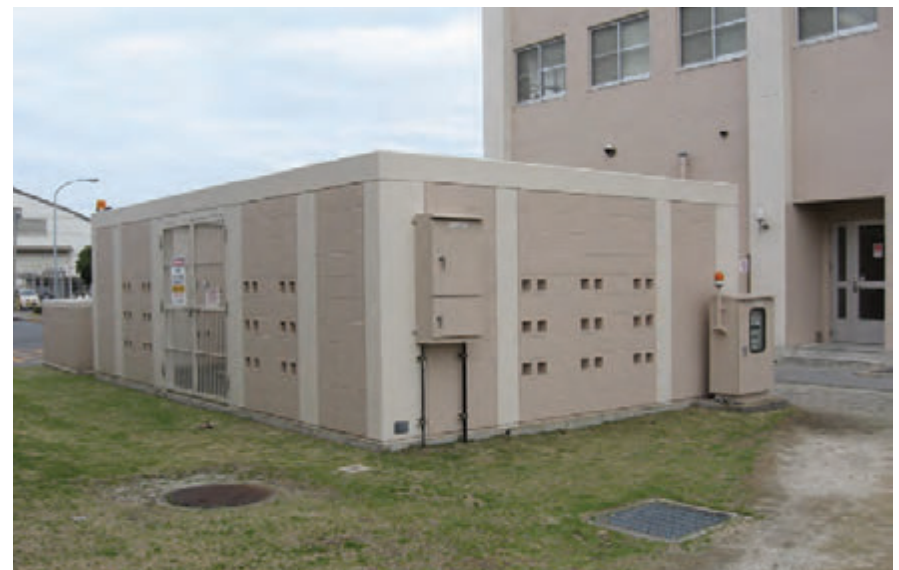
Screen wall enclosure that blends with the adjacent building architecture
