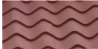
Concrete-formed simulated tile roofing
