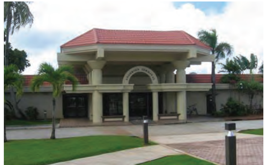
Monumental building entrance, out of scale with building façade
