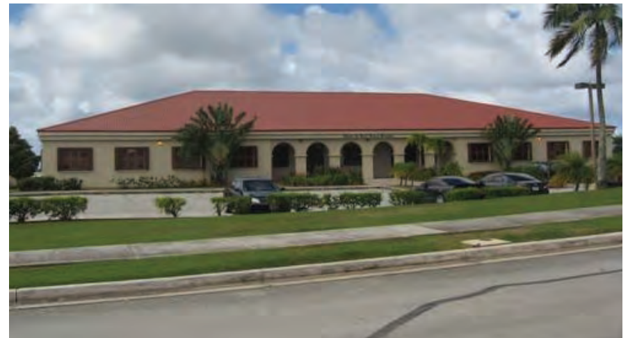
Rhythm of windows and arched entry openings provide balance to the building façade
