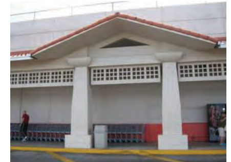
Latte stone pair supporting roof dormer
