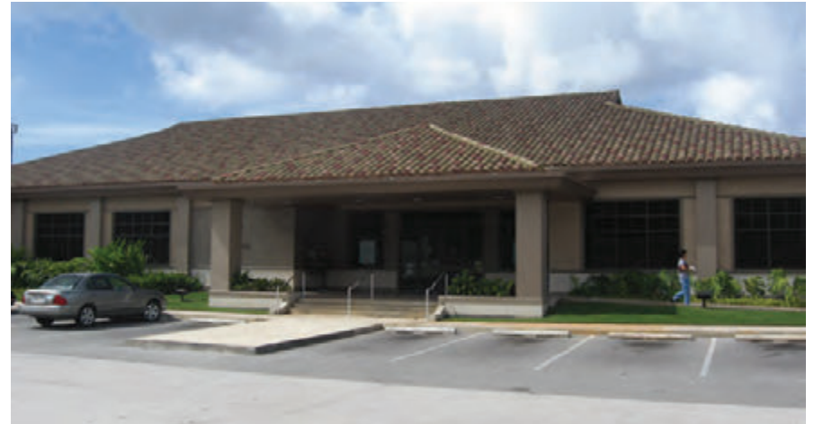
Textural quality provided by play of textured tile roof and articulated exterior walls
