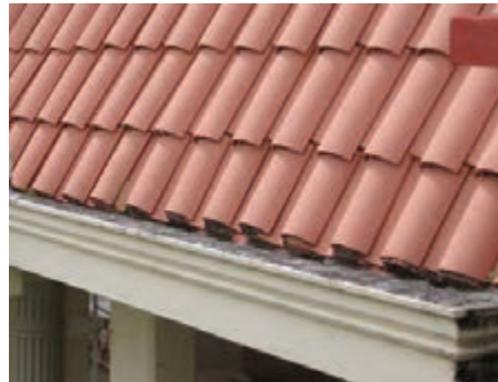
Concrete integrated gutter with simple fascia profile
