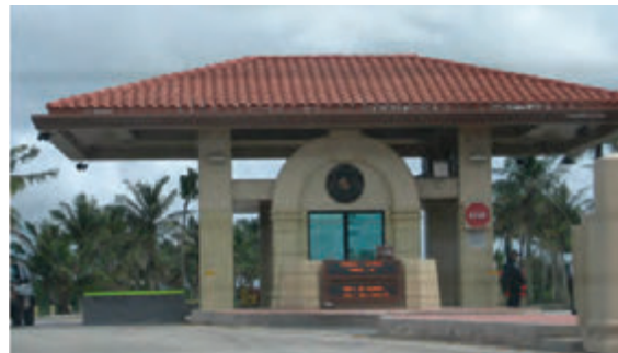
Andersen AFB entrance gate example
