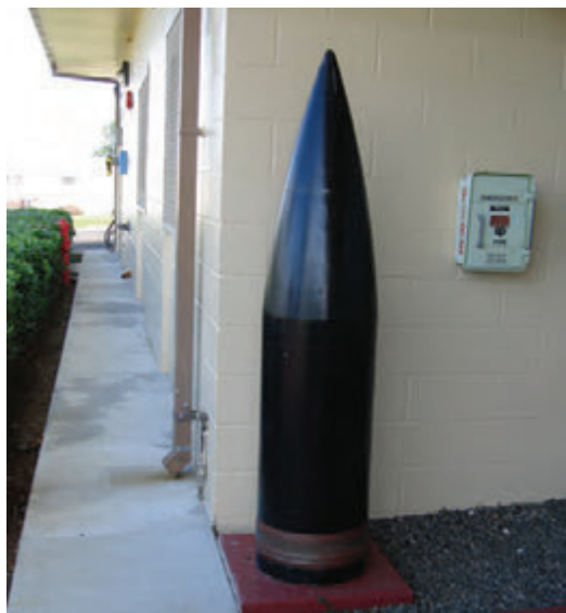
Concrete maintenance strip (Note: downspouts should not discharge at walkway)
