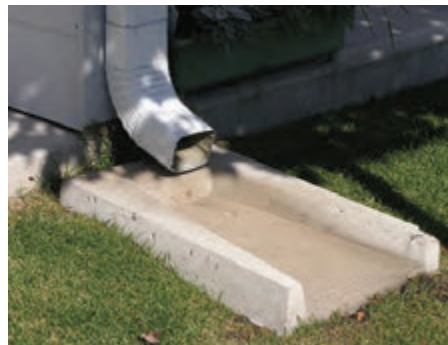
Elongated concrete splash block where downspout discharges onto unpaved areas
