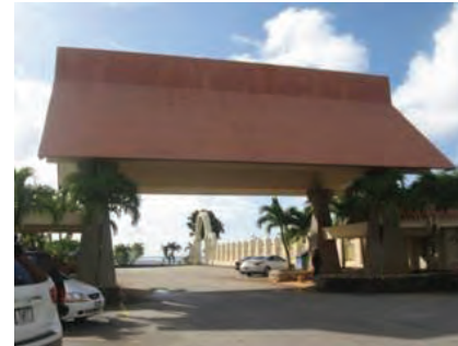
Double rows of Latte stones supporting roof structure
