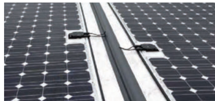
Low profile, BIPV solar modules for low slope roof applications
