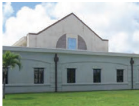
Example of base trim and profiled recesses
