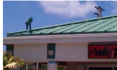
Concrete batten roof
