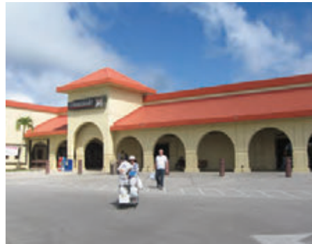
Portico entry connected to an arcade
