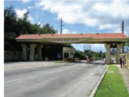
Literal and abstract use of Latte stone at entry gate
