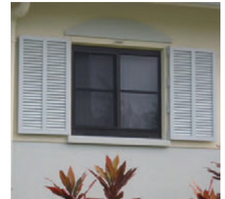
Colonial style (hinged) shutters with integrated polycarbonate protective covers on back side of shutter panels
