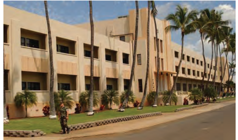
Rhythm expressed through regular bays, aligned openings, fenestration, and expressed structural columns
