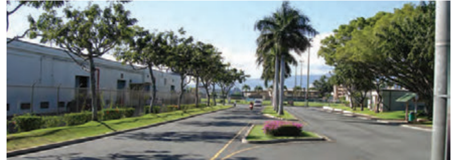
The roadway system is the major vantage point from which the installation is viewed; an attractive streetscape enhances the visual image of the installation
