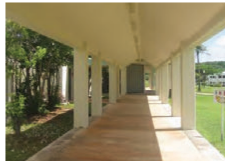
Covered walkway connecting buildings
