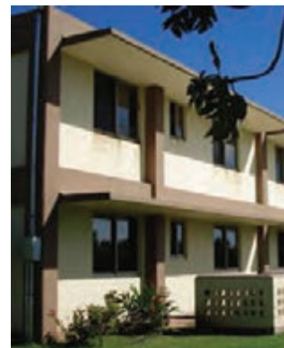
Concrete flat awning
