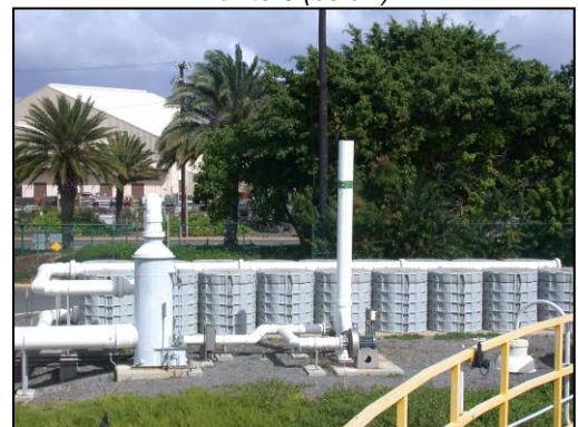
Headworks (above) with Odor Reduction Biofilters (below).
