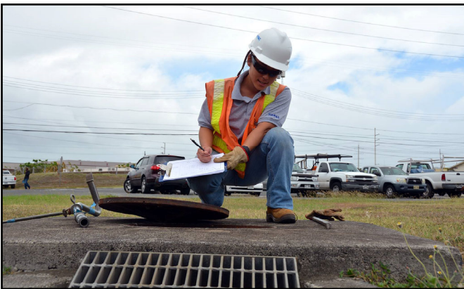
Figure 2: Inspection of a storm water drain inlet. (U.S. Navy photo by Denise Emsley)
