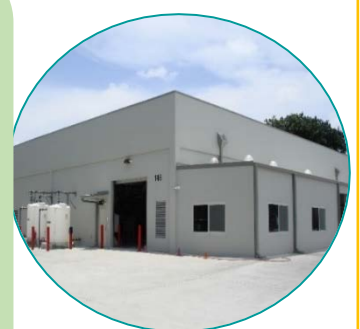
Figure 4. Main WTP at Cantonment
