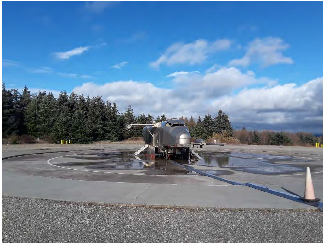
-Current fire training pit and mock aircraft (facing northwest)
