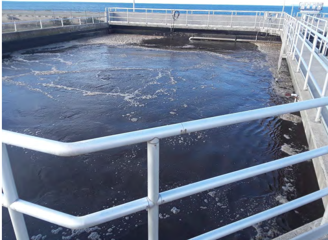
-Wastewater treatment pond (facing west)
