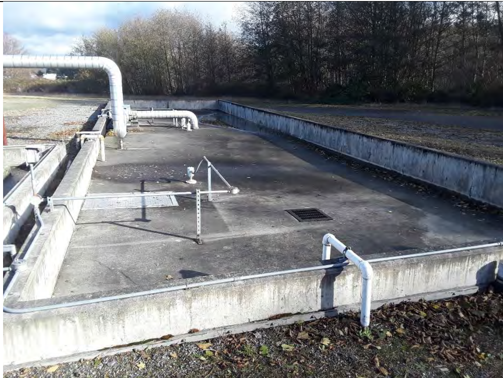
-Detention pond – water was stored here prior to entering oil/water separator (facing east)
