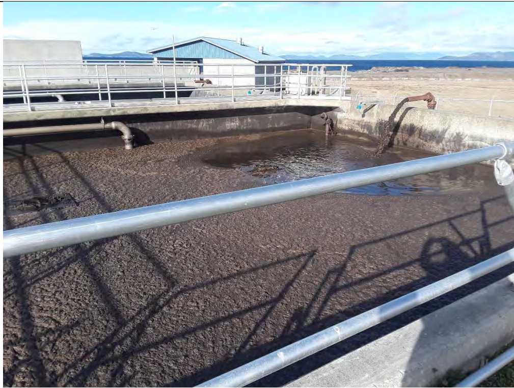
-Treatment pond (facing northwest)
