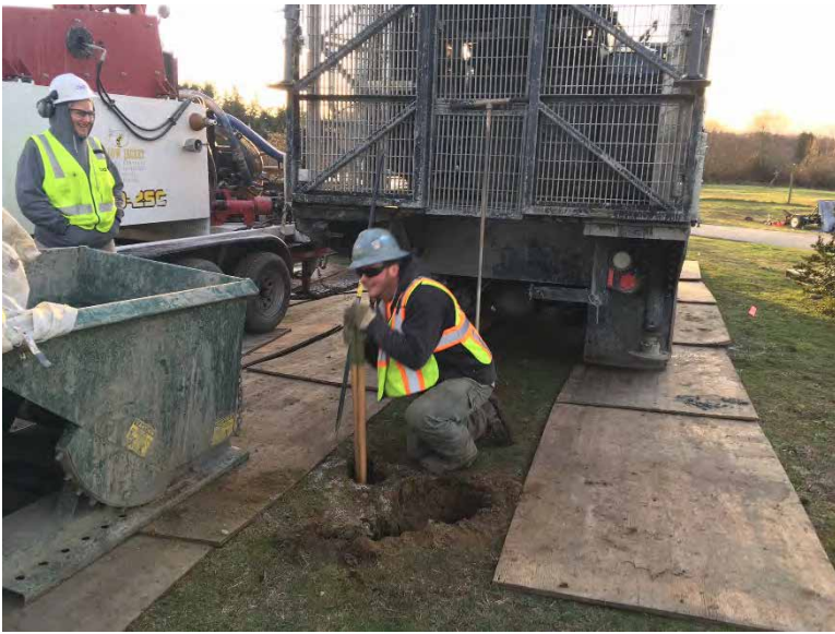
Photo 1. Overview of pre-drilling hand auger placement at boring location.
