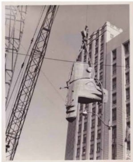
Thunderbird head being installed.jpg
