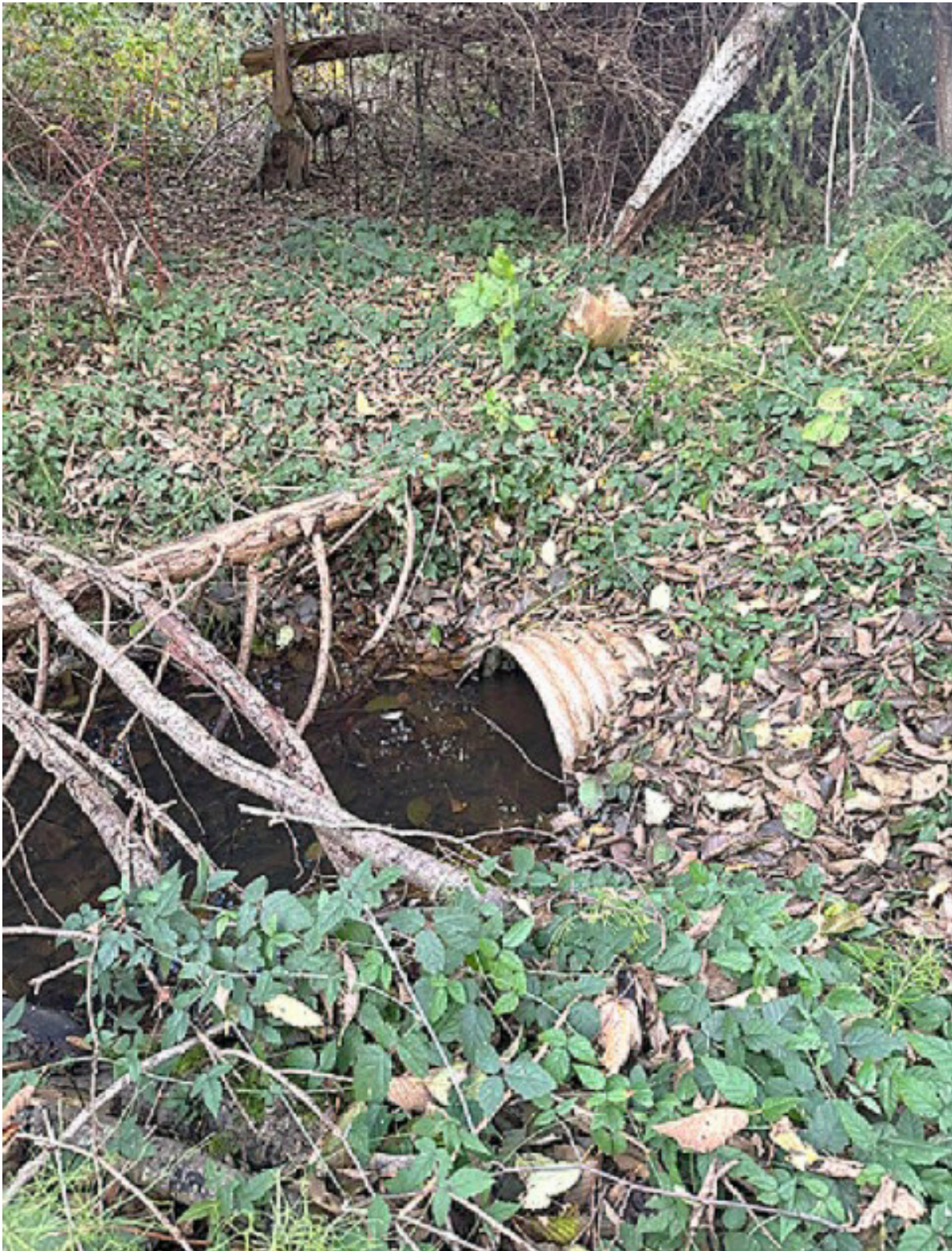
Figure 3-5 Existing Stormwater Outfall to Hayho Creek, West of Project Site
