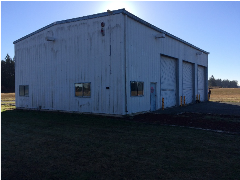
Building 2709 (facing southeast)
