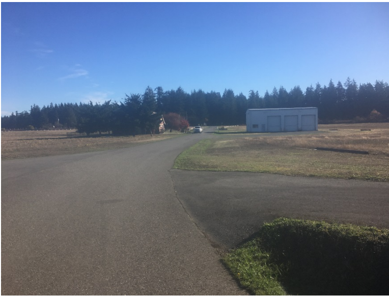
View of Fireman's Quarters and Building 2709 facing east.
