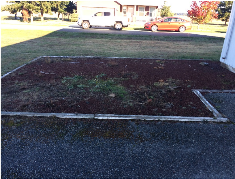
Gravel area (presumably wash pad) at the northwest corner of Building 2709
