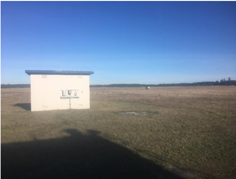
Facility 10 (Runway Lighting Vault)
