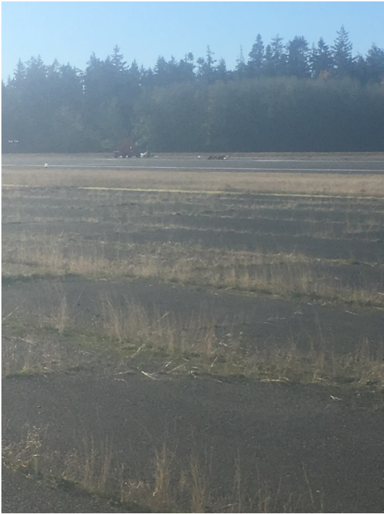
South end of runway (facing southwest)
