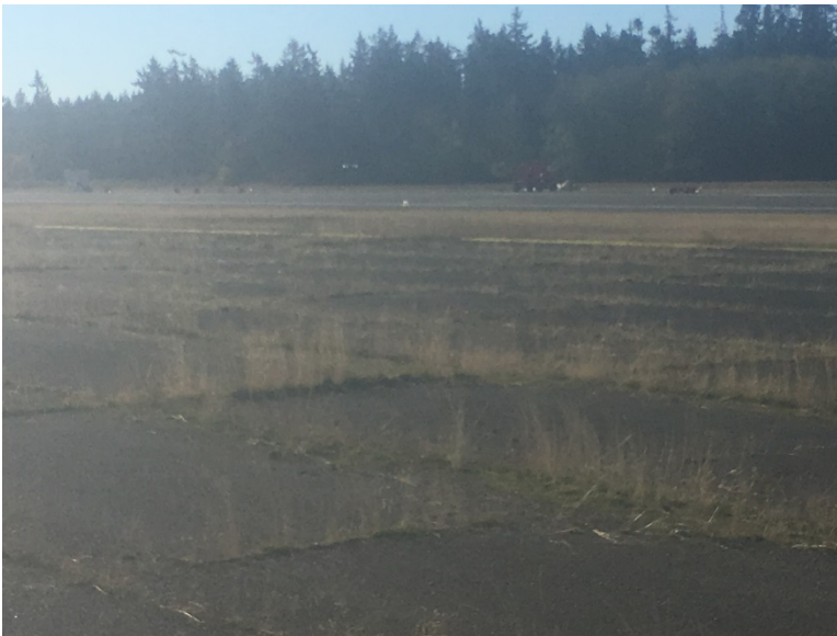
South end of runway (facing southwest)
