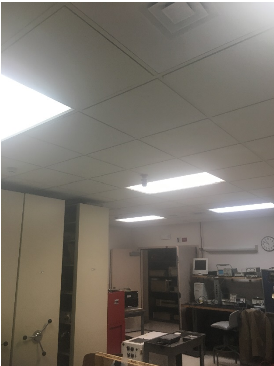
Halon fire suppression system in Building 2807
