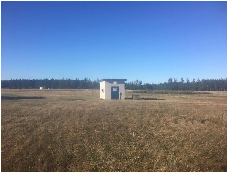
Facility 10 (Runway Lighting Vault)
