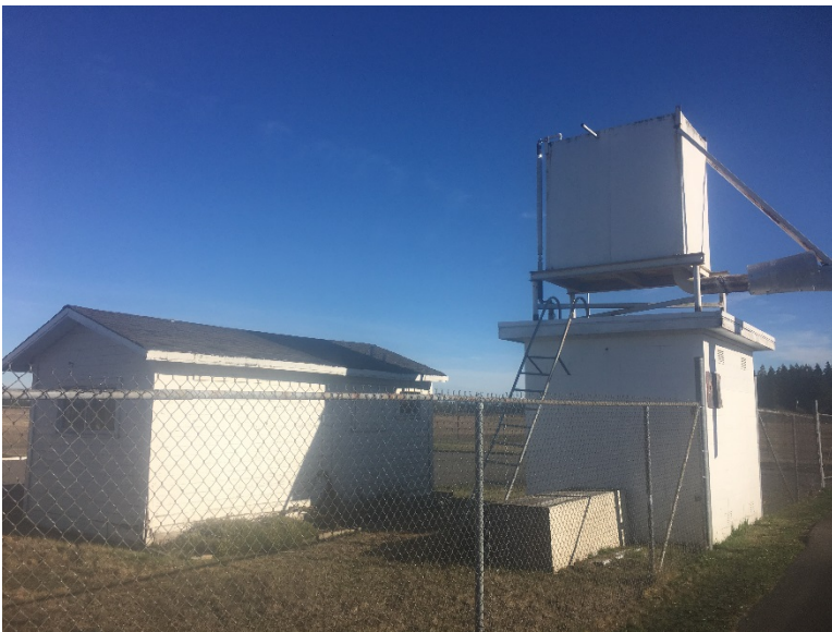
Facility 2 (Airfield Operations Building) (left) and Facility 11 (Potable Water Well Pump House) with PF Tank 11 on roof (right)
