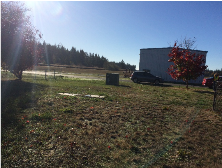
View of Building 2709 from the front (south side) of the Fireman's Quarters
