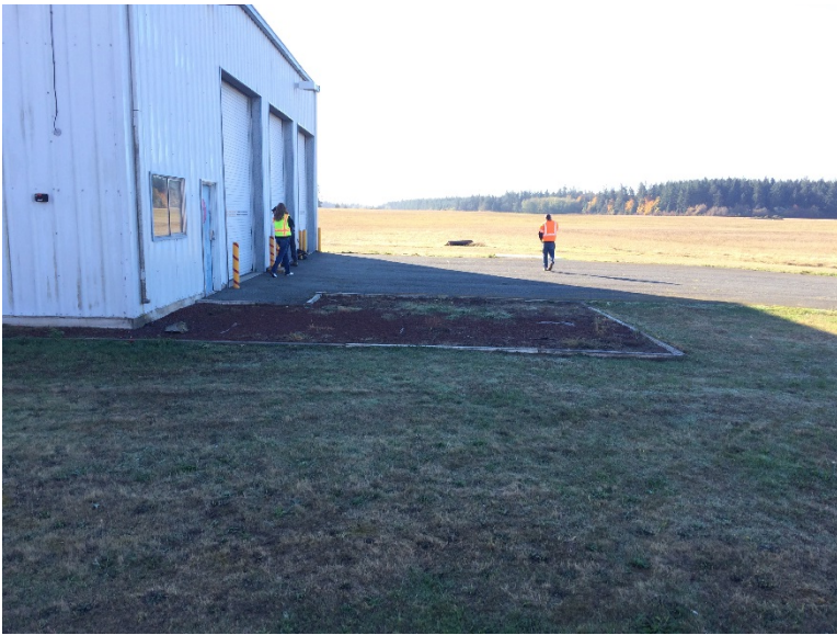
Building 2709 with west-facing bay doors and gravel wash pad (facing south)
