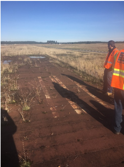
Possible old runway surface between current runway and taxiway
