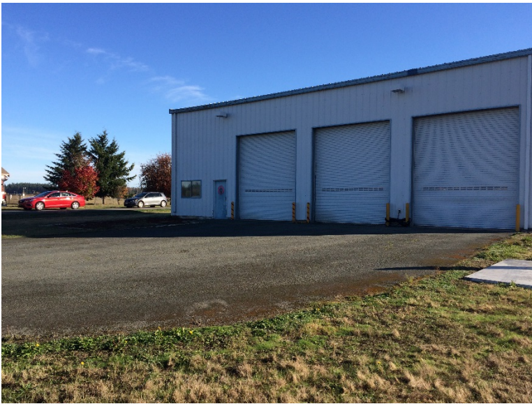
Building 2709 (facing northeast)
