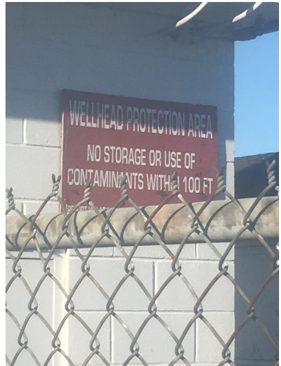
Wellhead protection area sign on Facility 11
