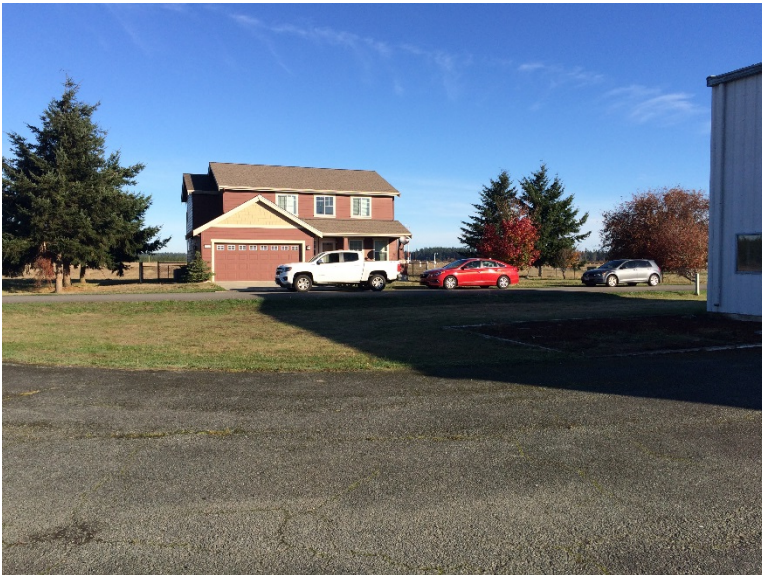
View of Fireman's Quarters from the driveway west of Building 2709
