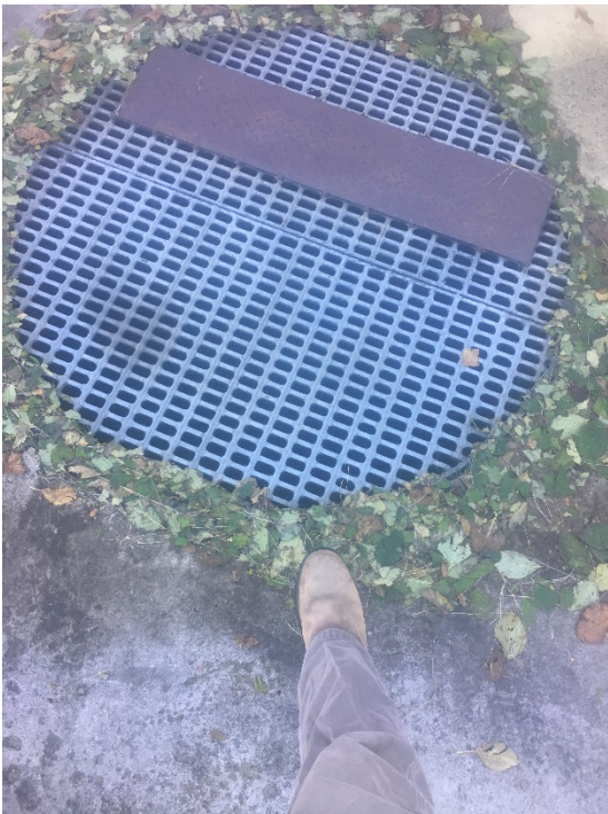
Stormwater inlet near the northeast corner of Building 2709
