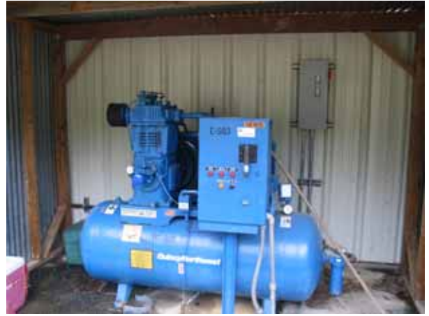
OU 1 (Site A) Treatment System Compressor
