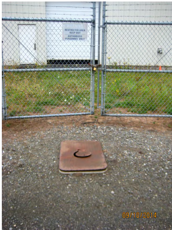
Damaged well vault cover at Site A
