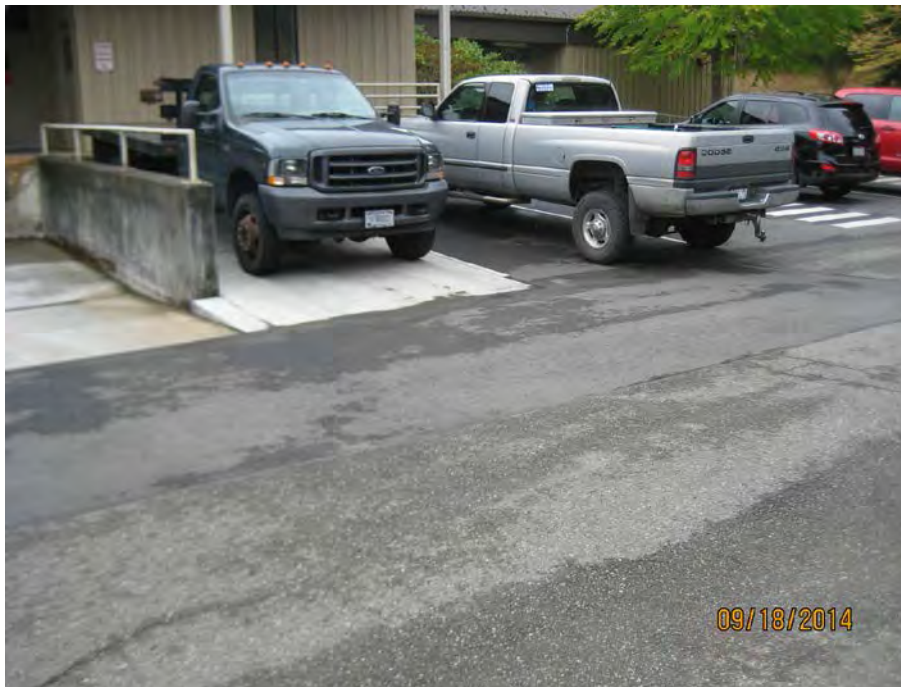
Cracked pavement observed at Site 10
