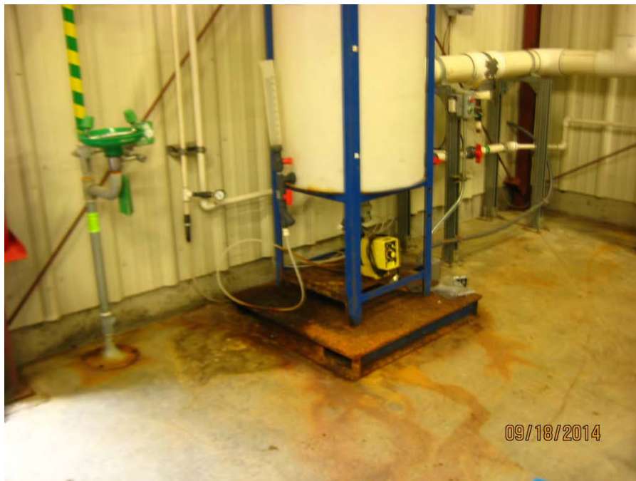
Corrosion observed inside Site A treatment system building
