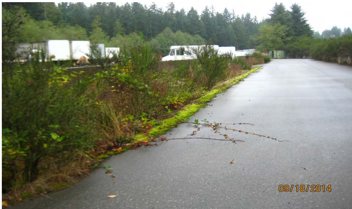
Vegetation observed growing in the drainage swale above the Site F infiltration barrier
