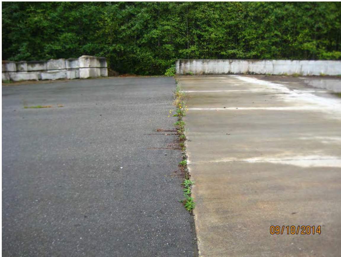
Vegetation growing in asphalt above Site F infiltration barrier
