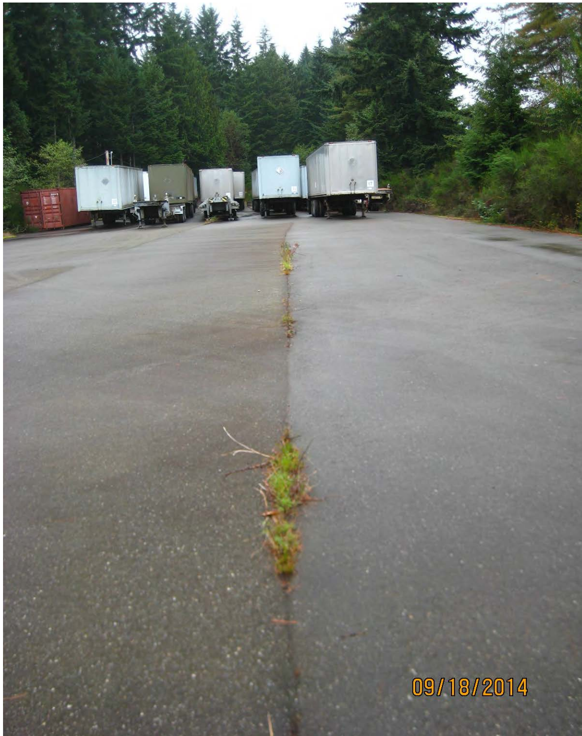
Vegetation growing in asphalt above Site F infiltration barrier
