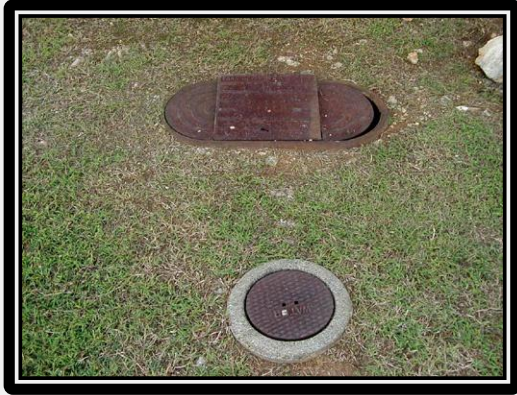
Water Meter Valve Box
