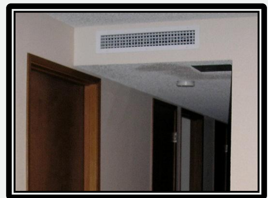
Wall Mounted Registers and Diffusers
