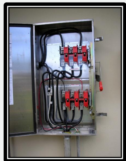
Stainless Steel Disconnect Switch
