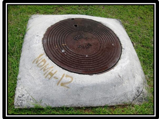
Storm Drain Manhole
