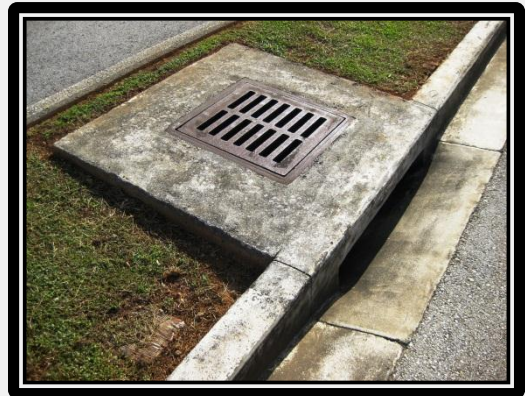
Combination Ground Surface and Curb Face Catch Basin
