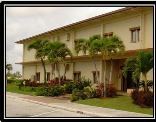
Low Slope Roof with Concrete Fascia
