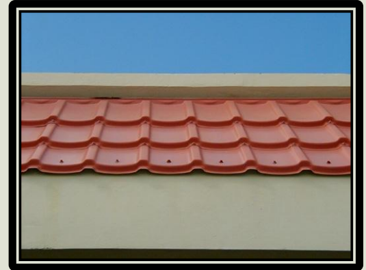
Existing Simulated Spanish Tile Metal Panels
