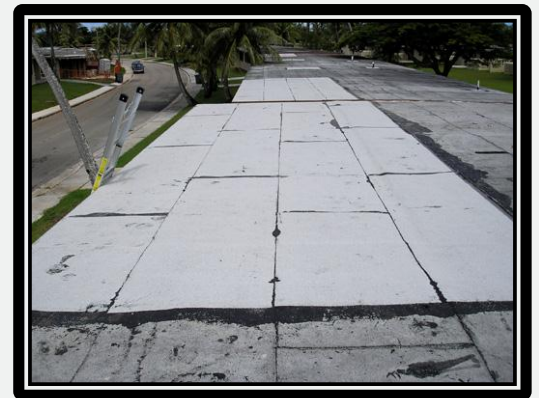
Existing Built-Up roofing System
