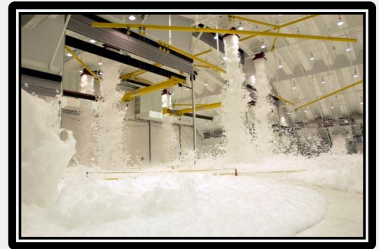
High Expansion Foam Fire Suppression System
